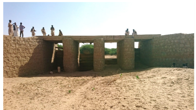
Photo 2 Intake of an irrigation canal in North Delta, GAS, Kassala
